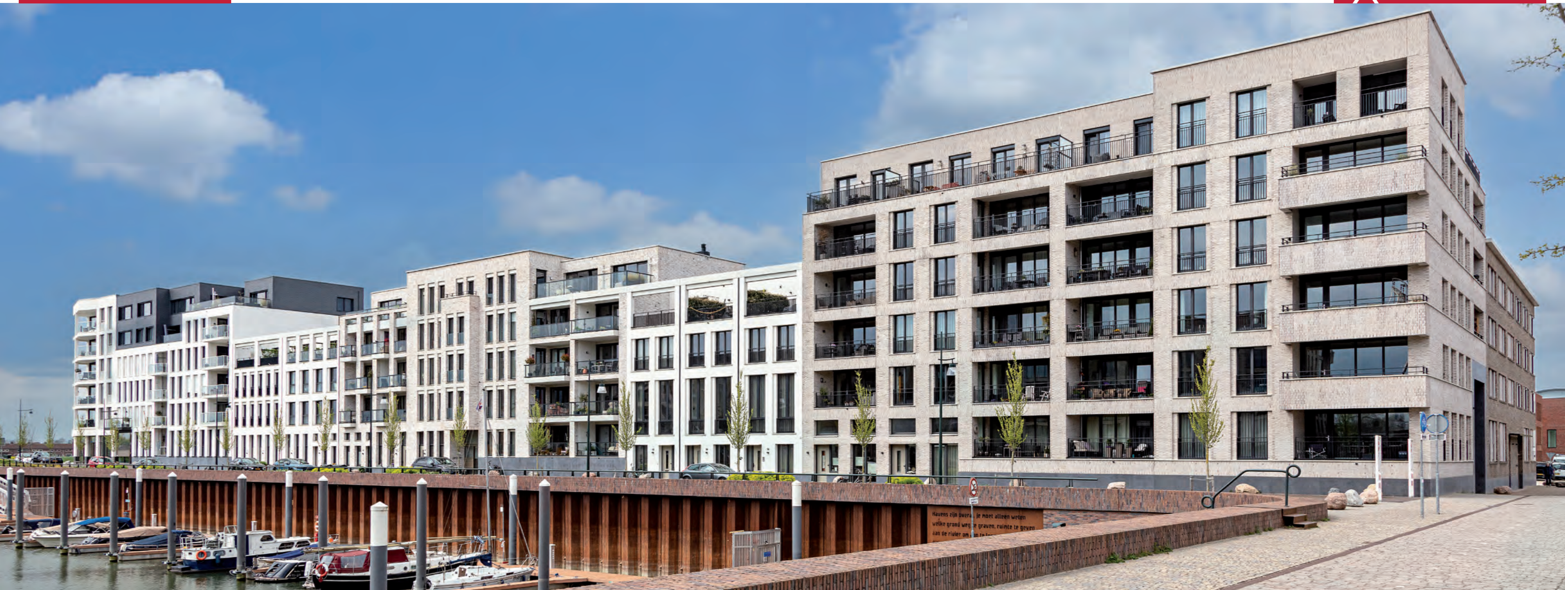
APPARTEMENTENCOMPLEX KADE NOORD, METIUSHOF, ZUTPHEN
